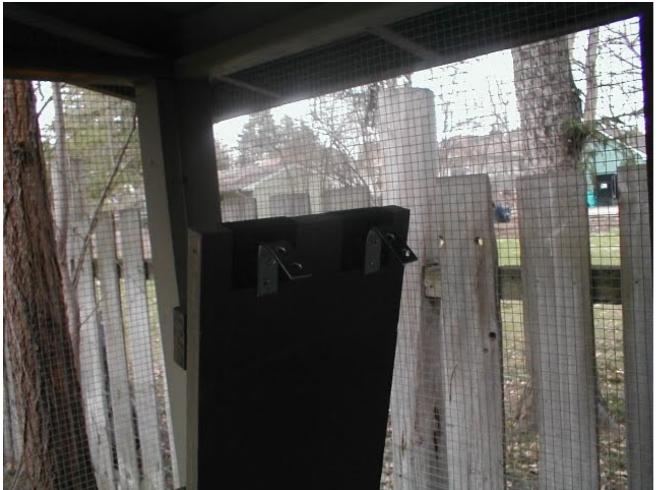
Corner braces on the bottom of the ramp fit into the slot below the ramp door.
