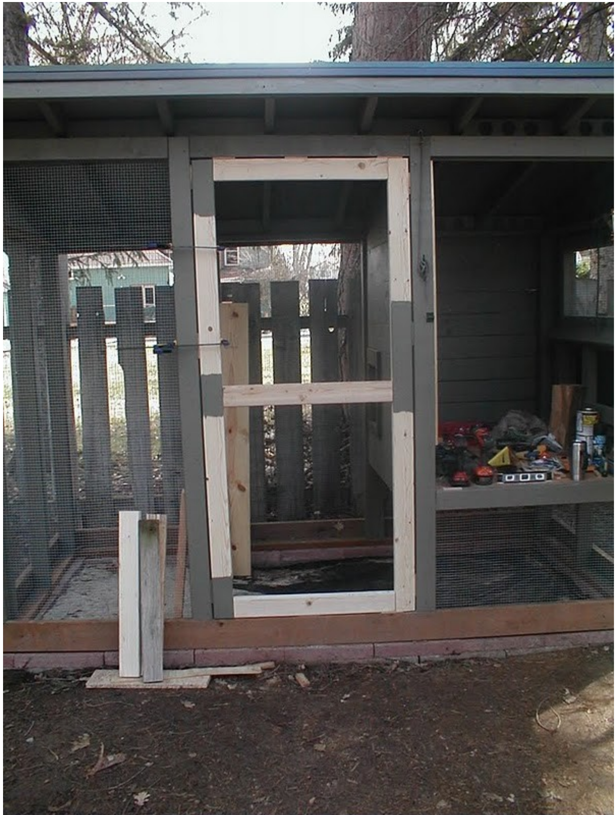
This door was built with the same shim/build-it-in-place approach.
