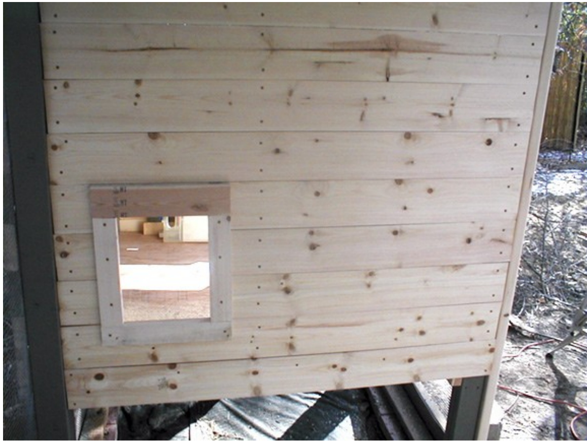
Framed the outside of the guillotine door both to make it sturdier and for looks.
