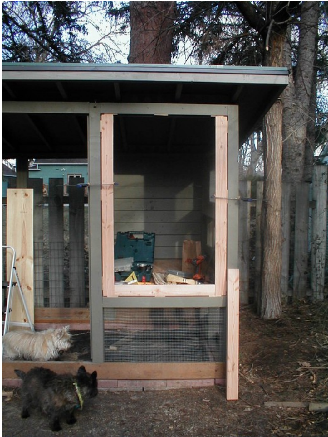
Building inspectors at work. Clamps hold the vertical lumber in place while I'm fitting it.
