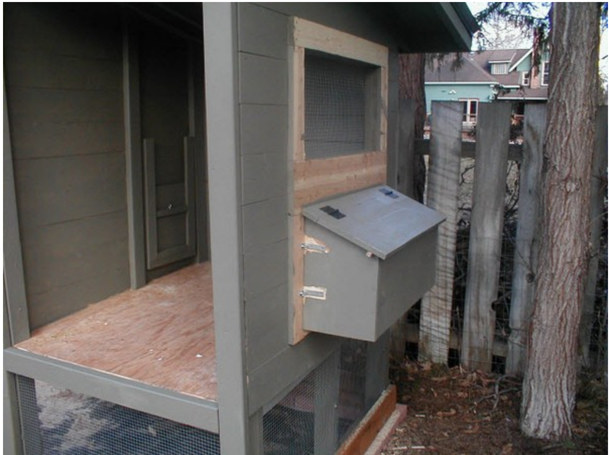
Framed the outside of the windows and nest box openings.
